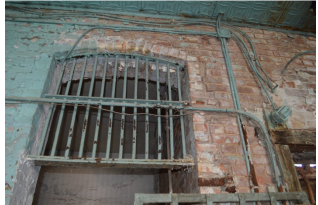
Figure 31: View of abandoned wires, conduits & junction boxes.
