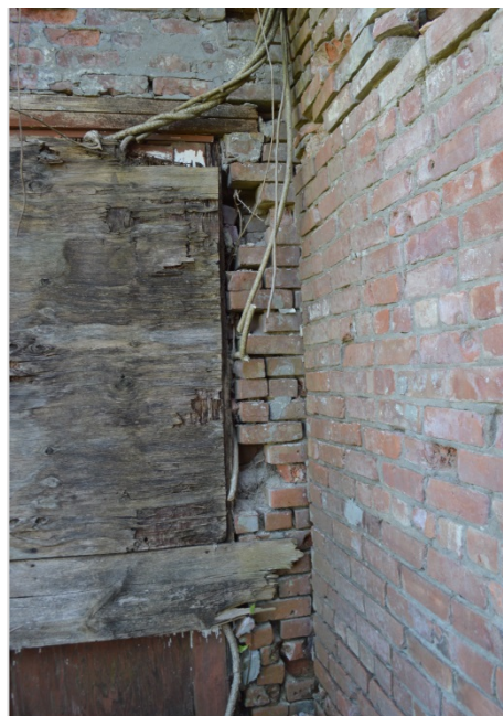
Figure 4: Detail of mortar & brick washout on inside corner of rear wall.
