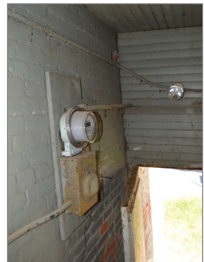
Figure 30: Electric meter & fuse box.
