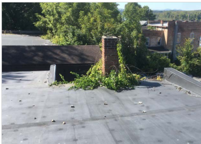
Figure 11: Roof from north side showing vegetation growing on rear chimney parapet walls.
