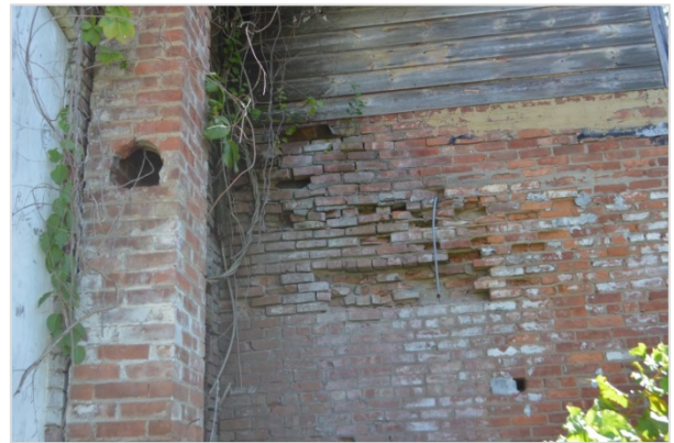
Figure 5: Loss of brick on west wall of south ell.
