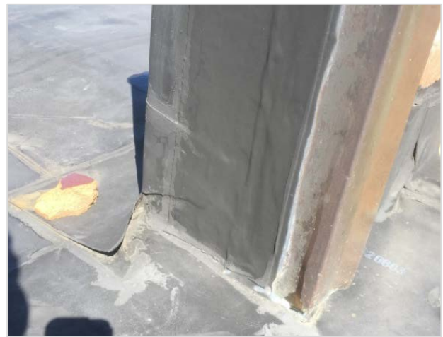
Figure 12: Detail of EPDM flashing up against parapet. Note lifted seam.
