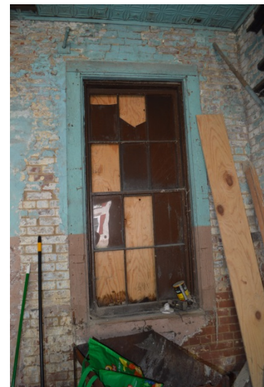
Figure 25: South wall of garage space showing remnant plaster under window.
