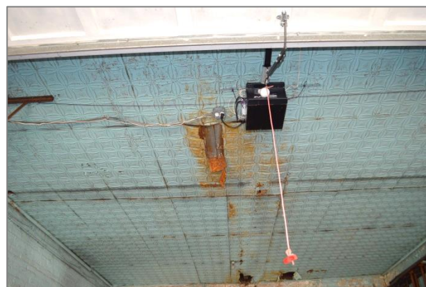
Figure 27: View of pressed tin ceiling in garage space showing rust at panel edges.
